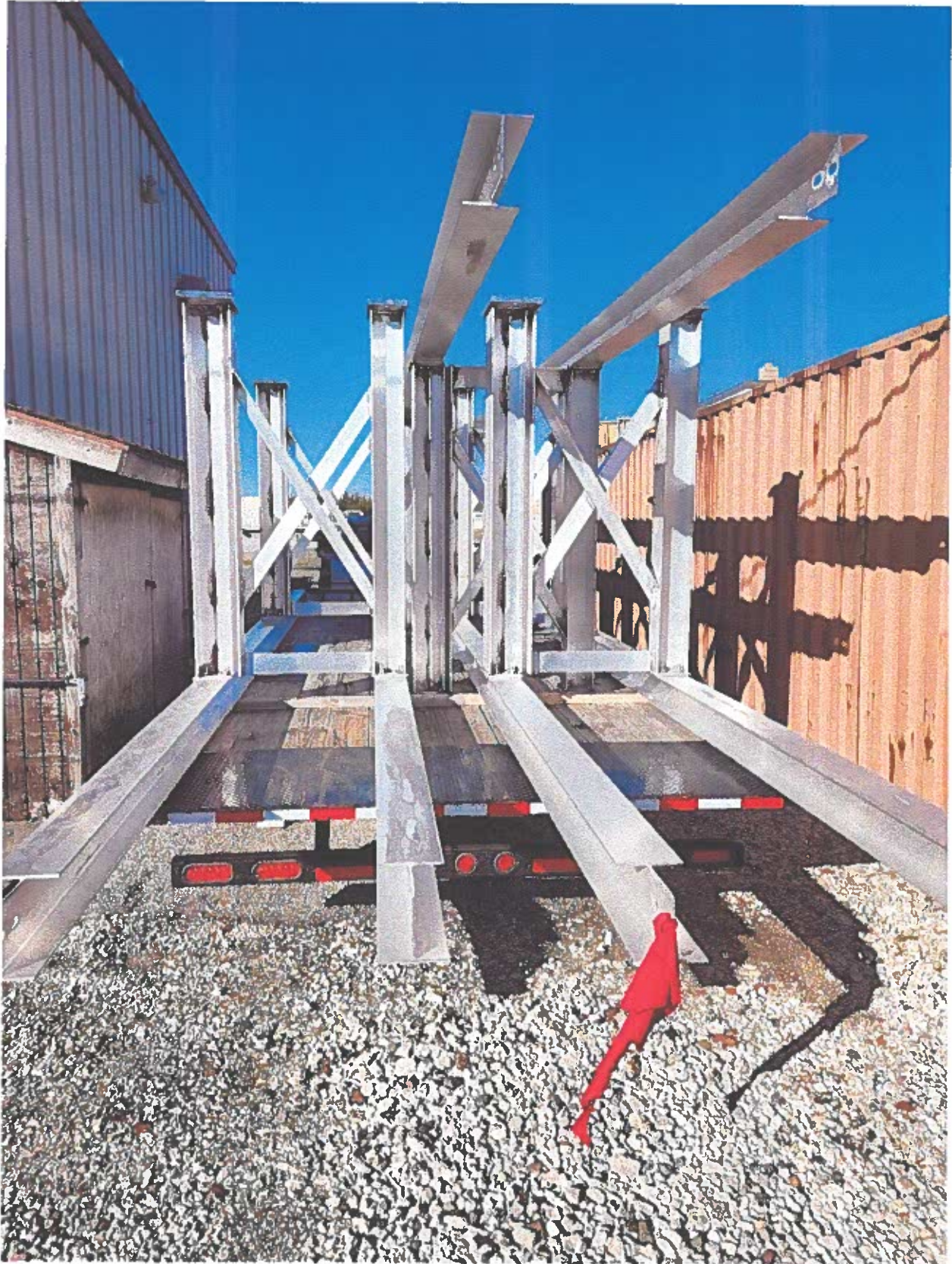
OC catwalk ready for installation
