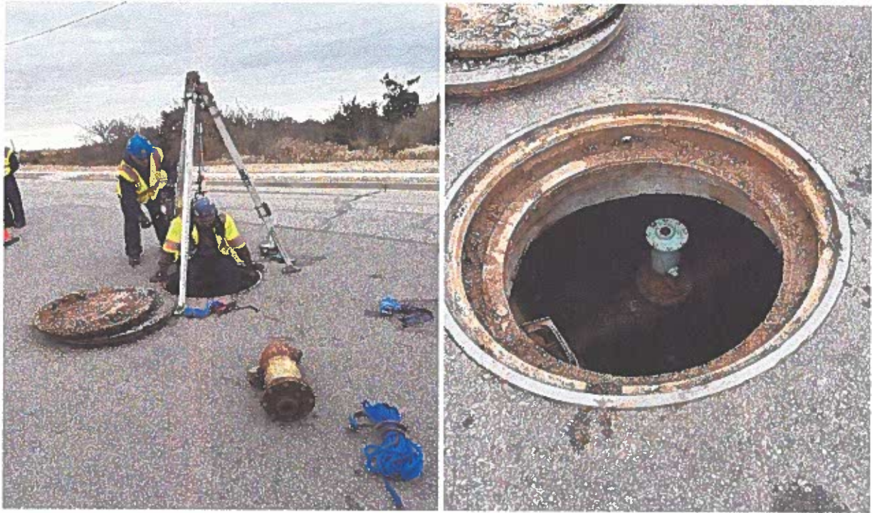
Oak Ave & Anglesea air release work
