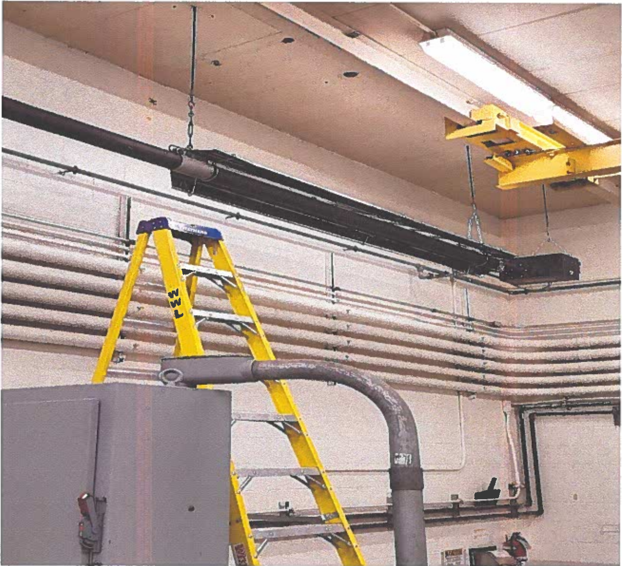
Spicer heater replacement
