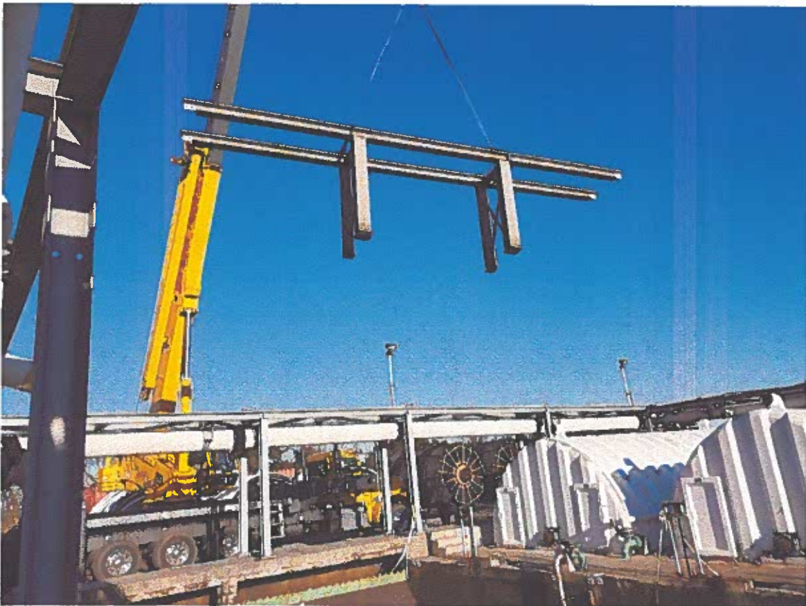
Crane removal of old RBC catwalks
