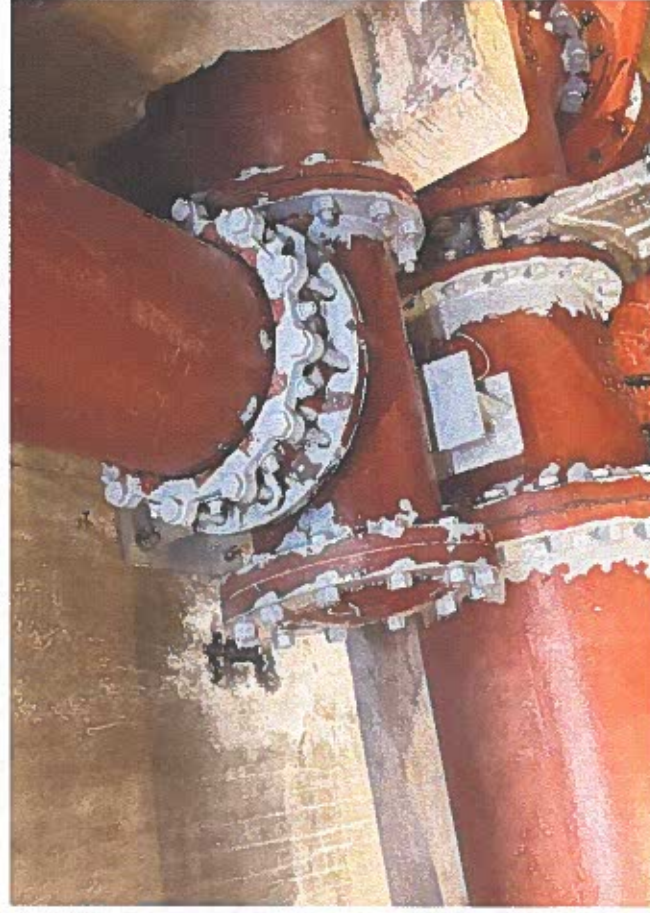
Painting being started, at hardware locations (12-14-23)
