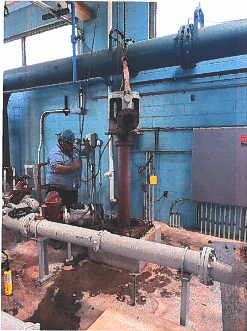
Hoisting/Removal of old pump
