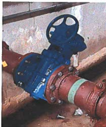
New Valve Installation
