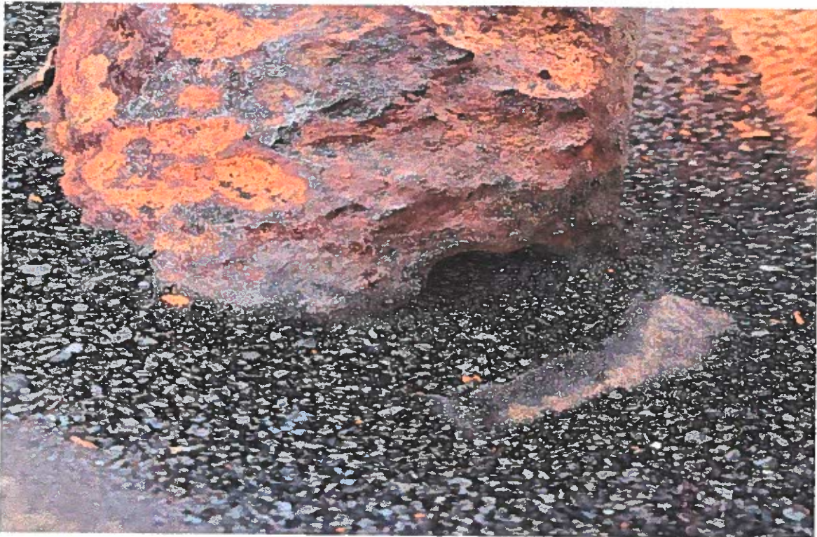
RBR Close up Corrosion
