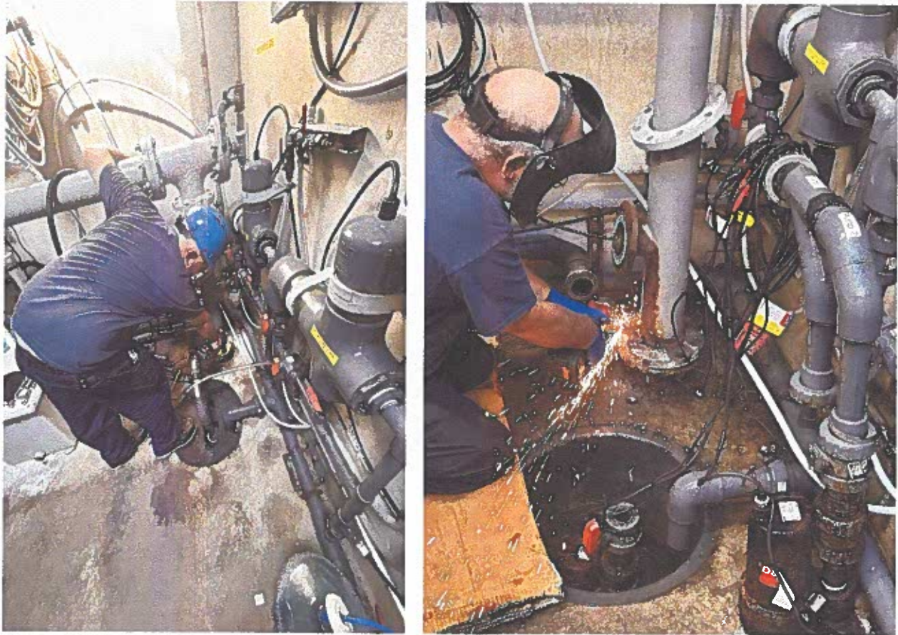
Sample pipe replacement.
