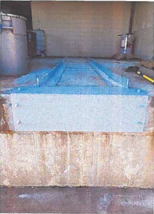
WW/L scum can guide rail installation
