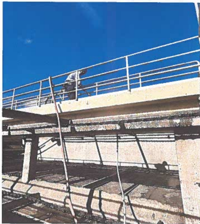
SMM clarifier maintenance and drive repair
