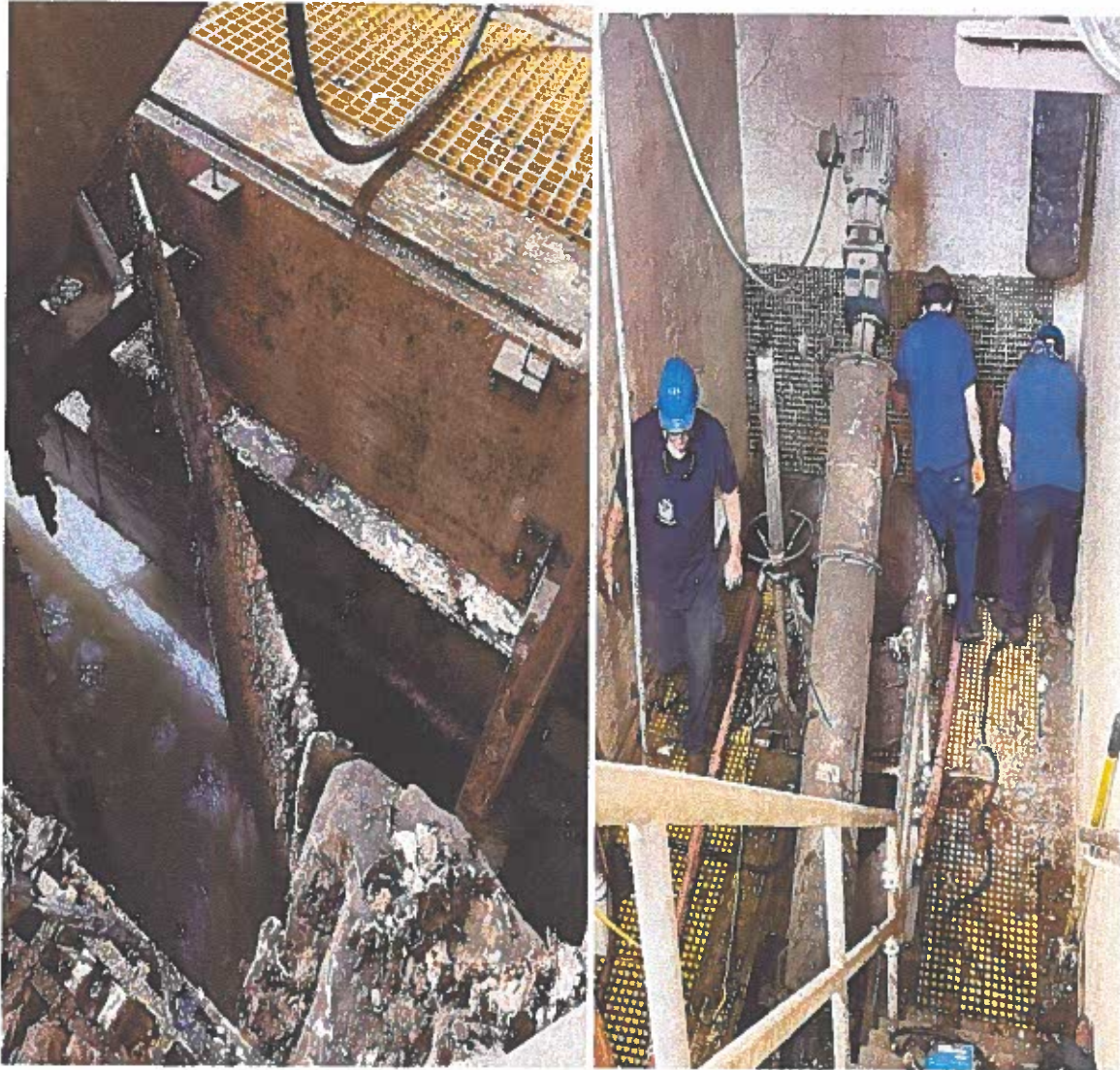
OC 3rd St wet well cleaning
