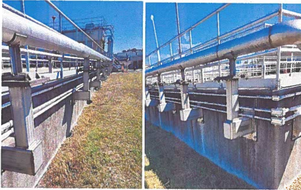
SMM Primary Scum Pit electrical installation
