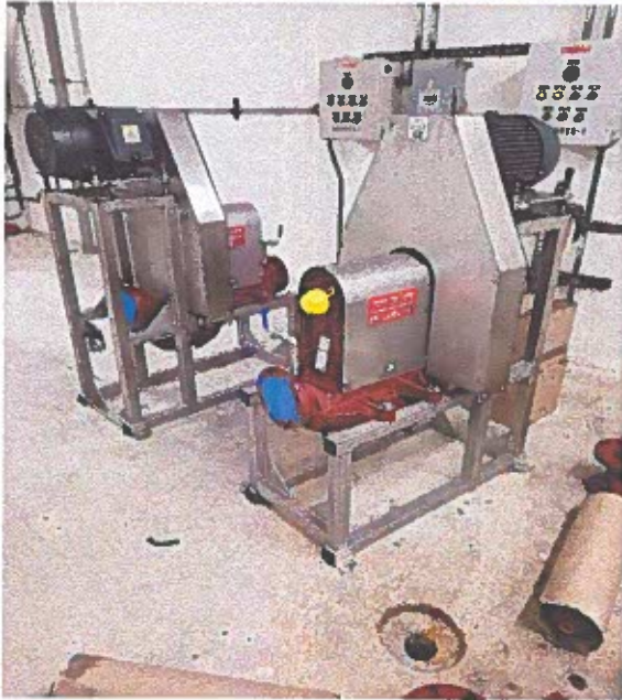
WW/L scum pump installation
