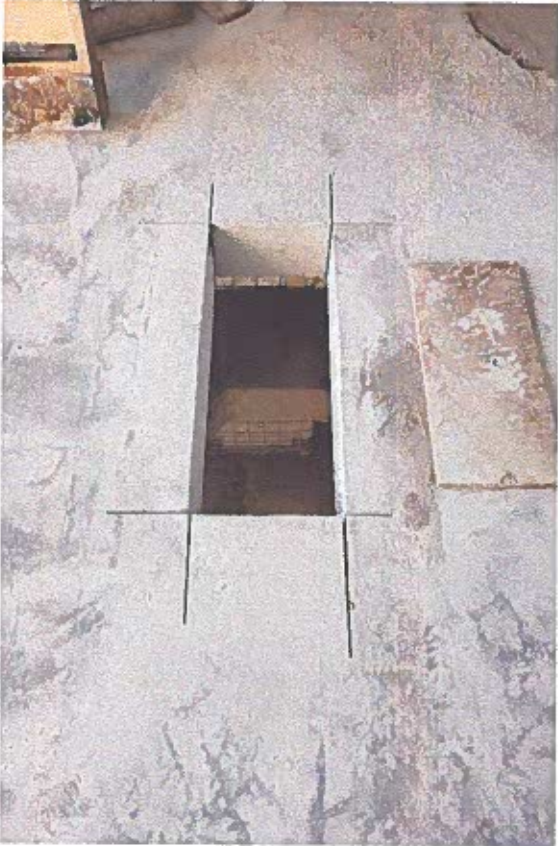
WW/L scum chute floor penetration
