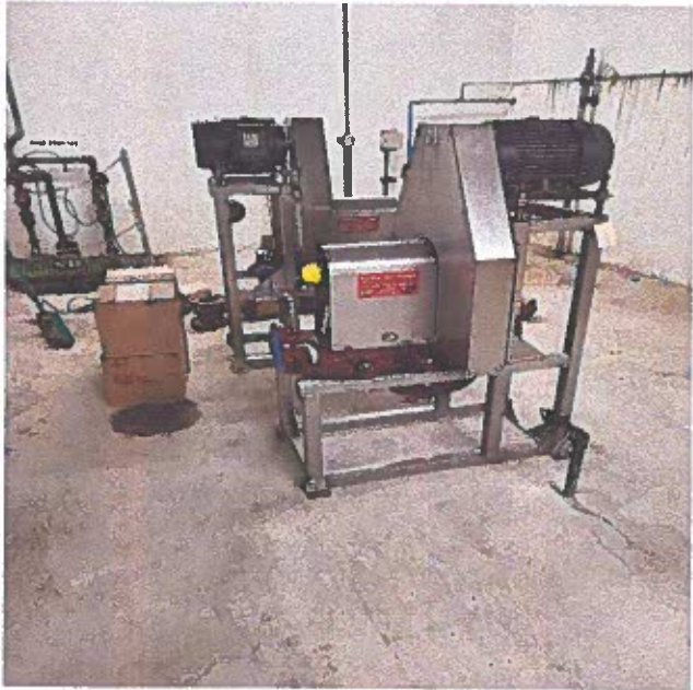
WW/L scum pump installation
