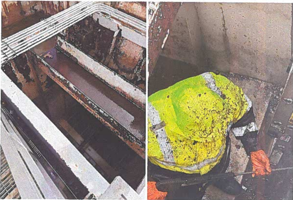
Powerwashing and surface preparation
