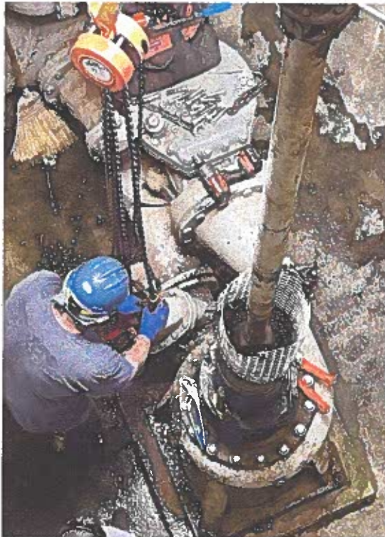
OC 3rd St valve replacement
