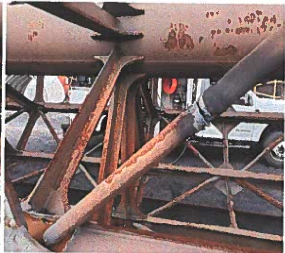
RBR support corrosion
