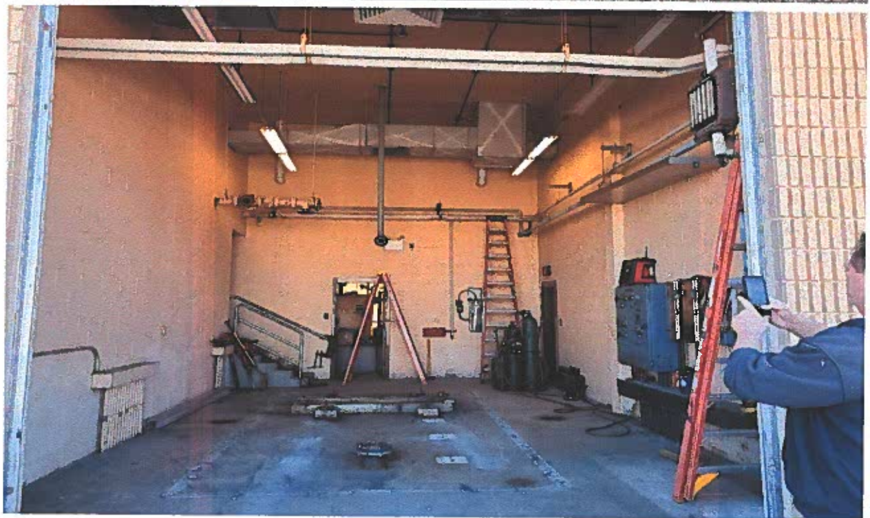
SMM Scum Concentrator demolition
