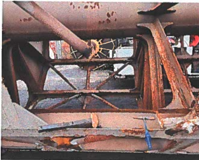
RBR support corrosion
