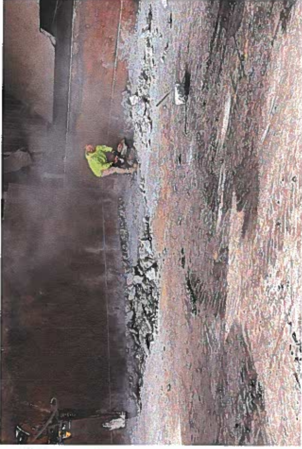
Saw-cutting to establish removal depth (10-18-22)
