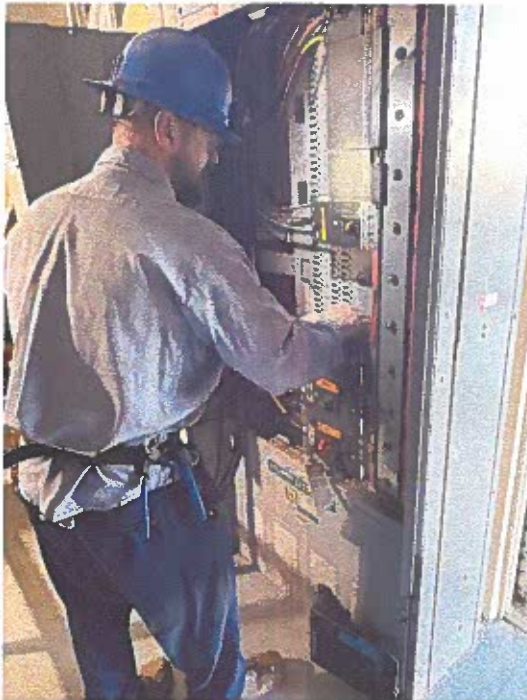
Paul Larsen, Plant Electrician
