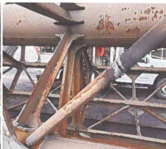
RBR support corrosion
