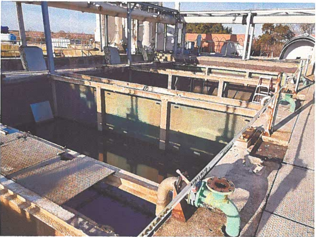
Aluminum catwalks being readied for demolition
