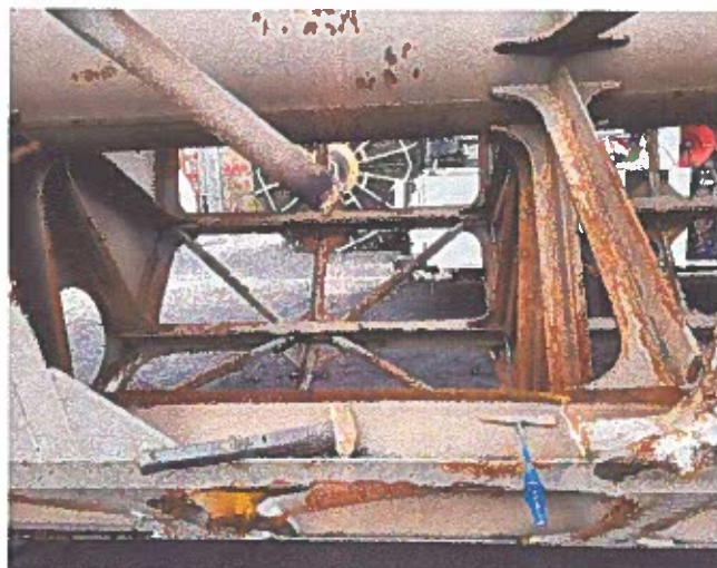
RBR support corrosion
