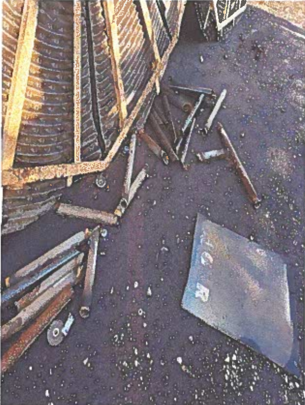
RBR old cross members removed
