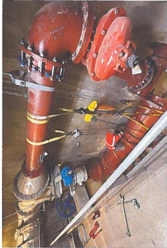
New discharge line manifold piping (11-13-23)
