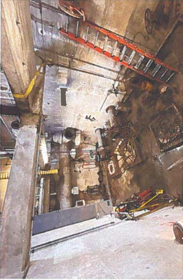
Demolition of existing piping (10-26-23)
