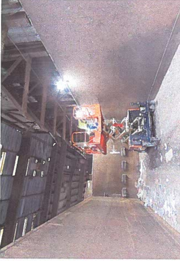
Installing supplementary support steel and anchors (1-19-23)
