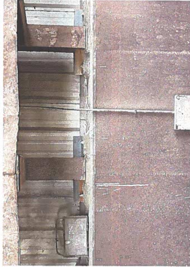
Installing supplementary support steel and anchors (1-19-23)
