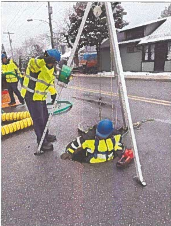
Cape May Air Release Inspections
