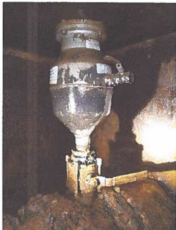
Cape May Air Release Inspections
