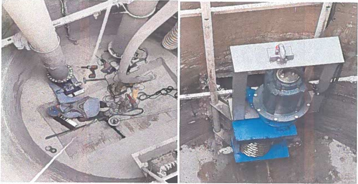
46th Street Pump Station pump and grinder installation
