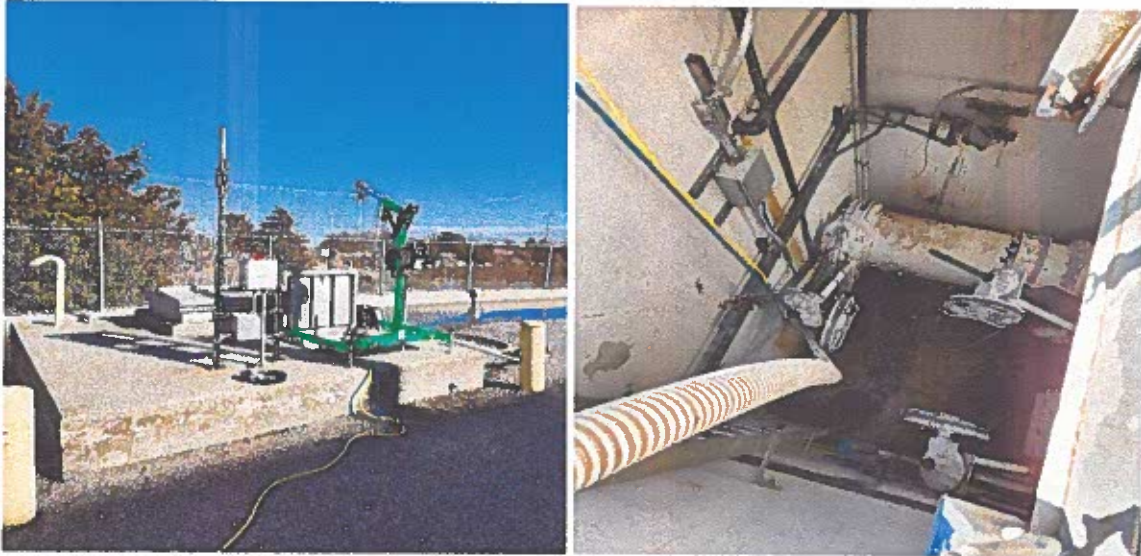
Effluent Vault sump pump repair
