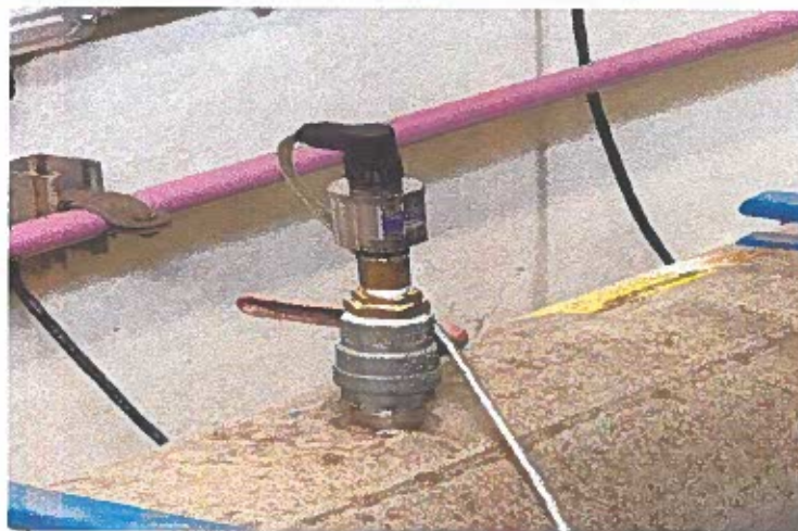
RWBR VFD install and pressure transducer move
