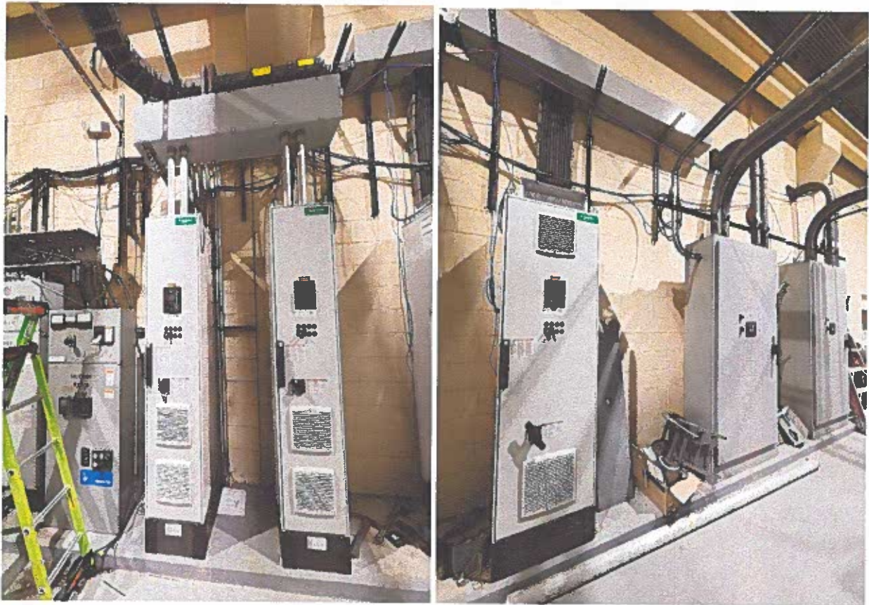
WW/L effluent pump VFD installation
