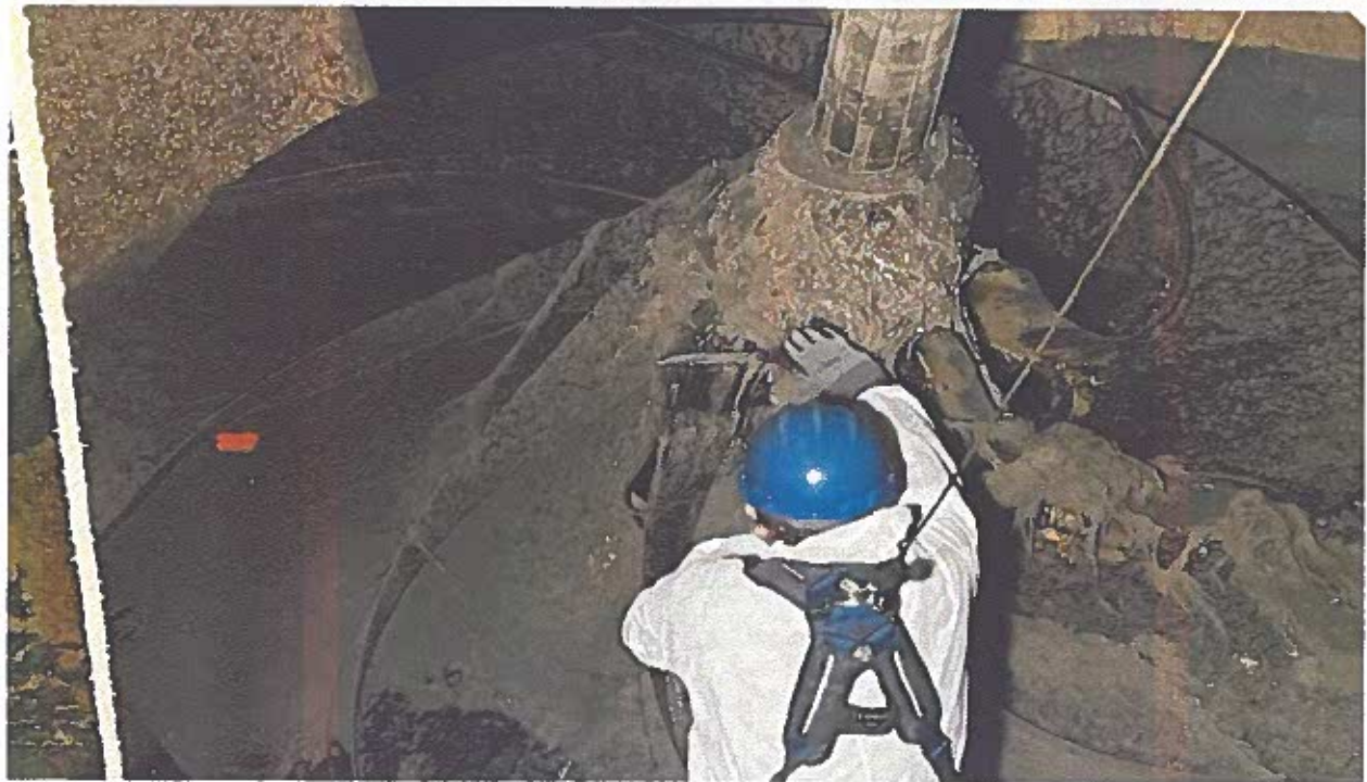
Sludge storage tank mixer cleaning
