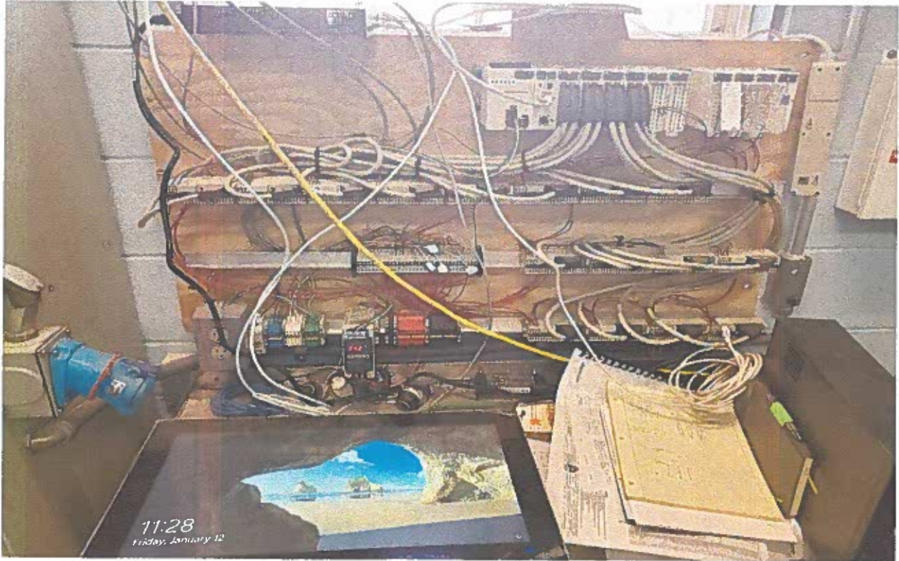
Madison Ave Pump Station SCADA installation temporary PLC
