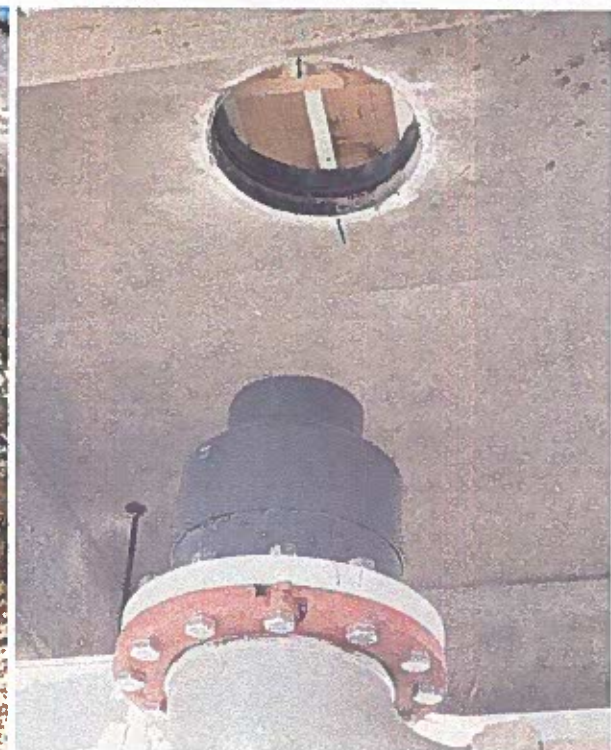
Clockwise from the top left - WW/L piping connections for the scum concentrator unit, SM/M core drilling wall penetration, SM/M underground scum system piping, and WW/L floor penetration core drilling
