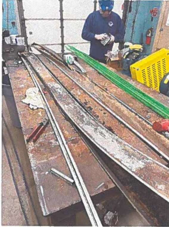
Fine air diffusers being rebuilt
