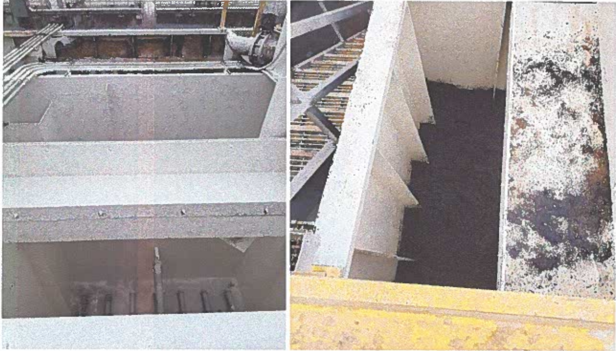
Final coating of filter cells and media installed
