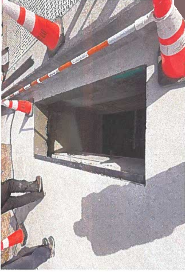
Final Clarifier cut complete (2-16-24)
