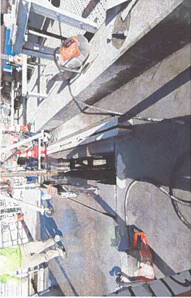
Removing Clarifier cut in segments (2-7-24)
