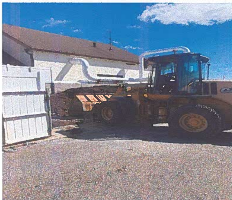
39th Street Pump Station Biofilter excavation
