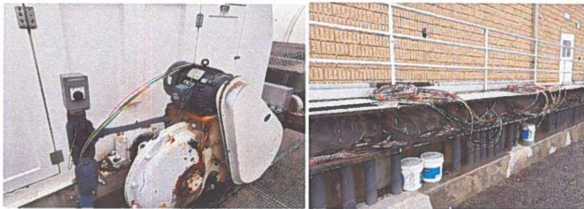
RBC wiring installation
