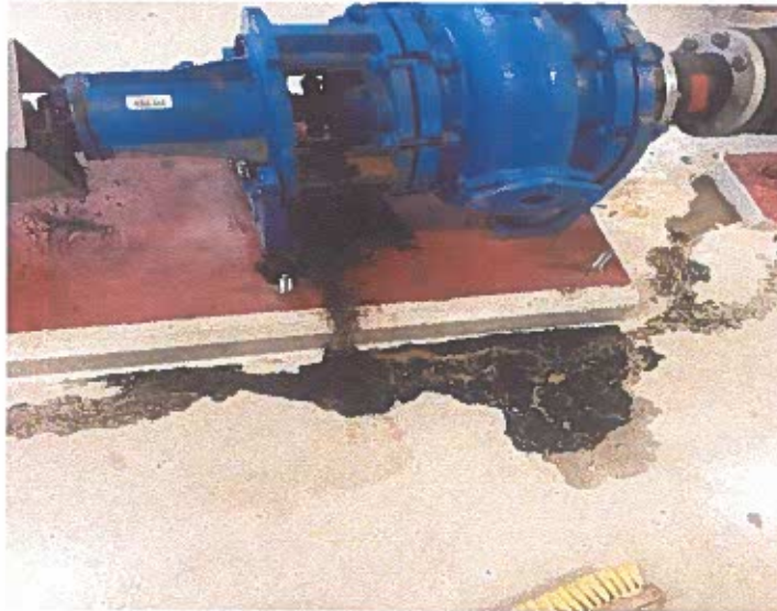
Primary sludge pump #2 packing repair
