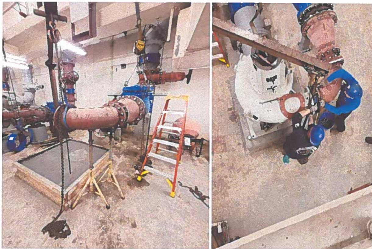
Spicer Ave pump station pump, piping and appurtenance installation
