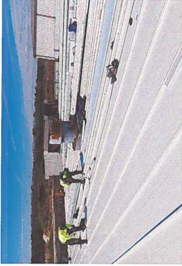
Fastening new roof panels (3-19-24)
