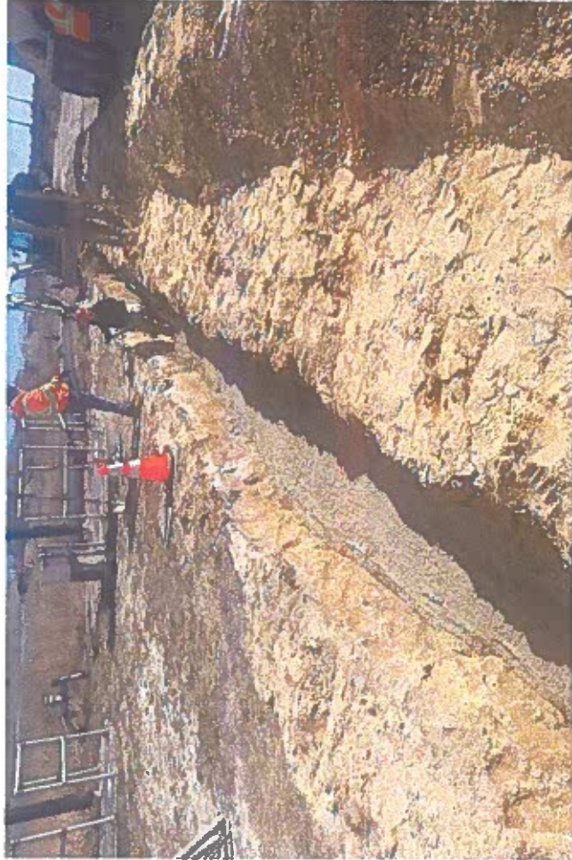
Concrete encasement (3-1-24)
