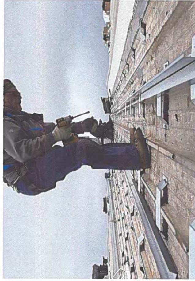
Inserting insulation into roof panels.
