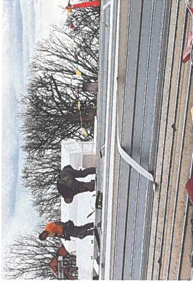
Inserting insulation into roof panels.
