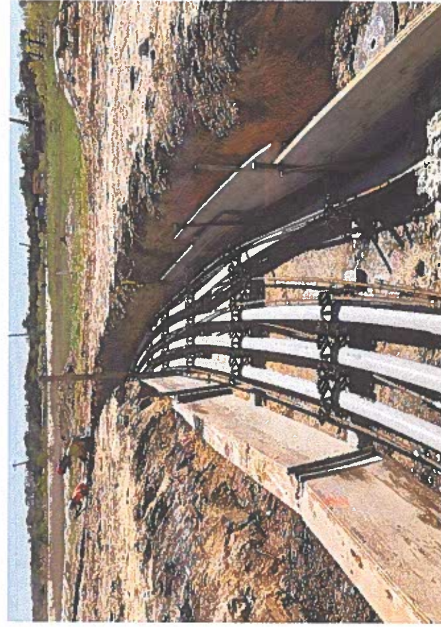
Conduit risers at backboard (4-15-24)
