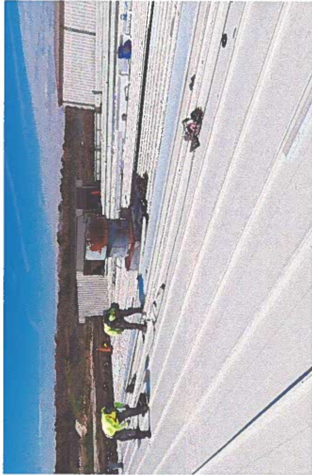
Constructing a new curb at the roof fan.
