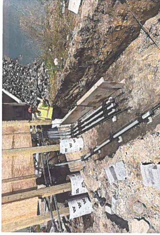
Conduit risers at backboard (4-15-24)
