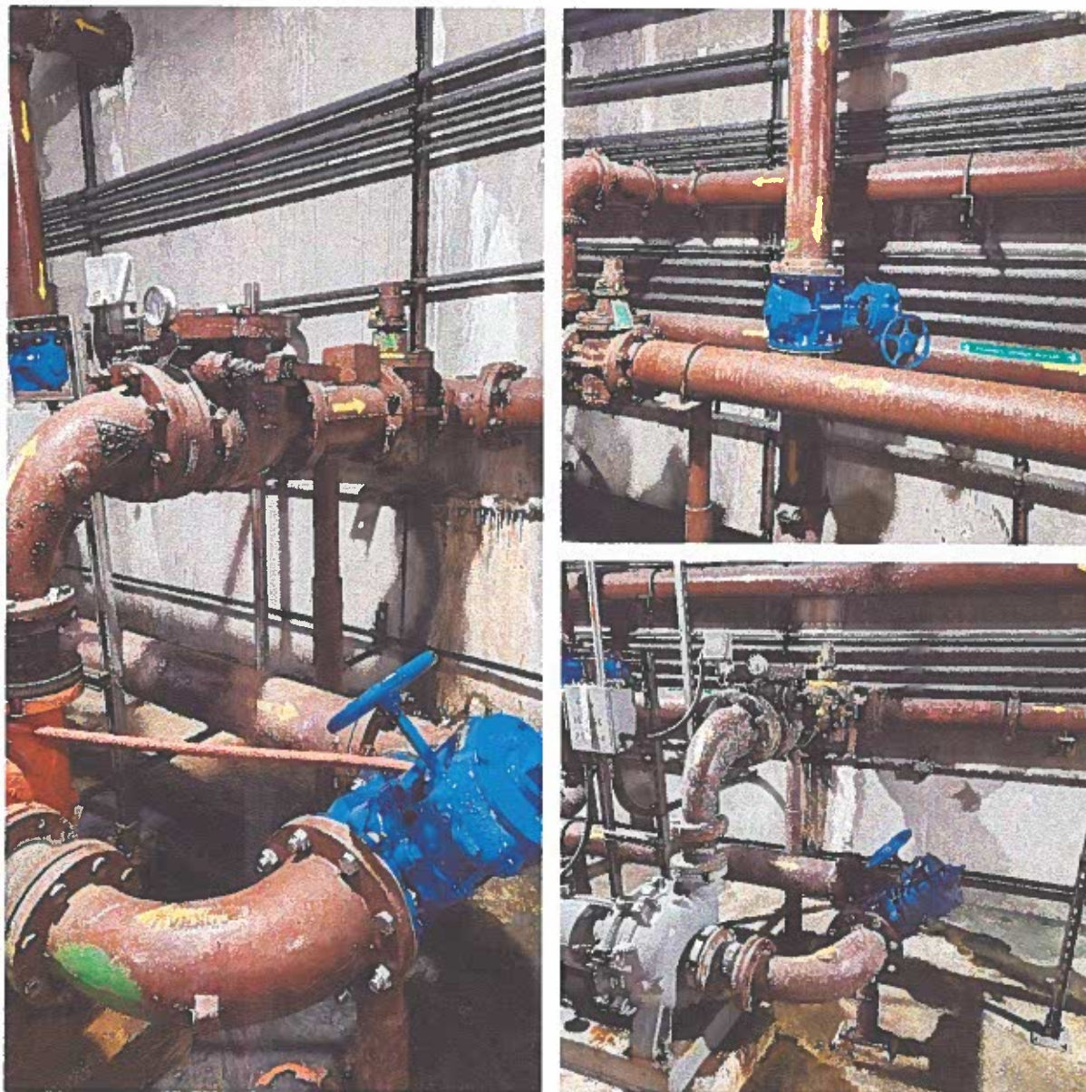
Valve replacement on the sludge waste piping
