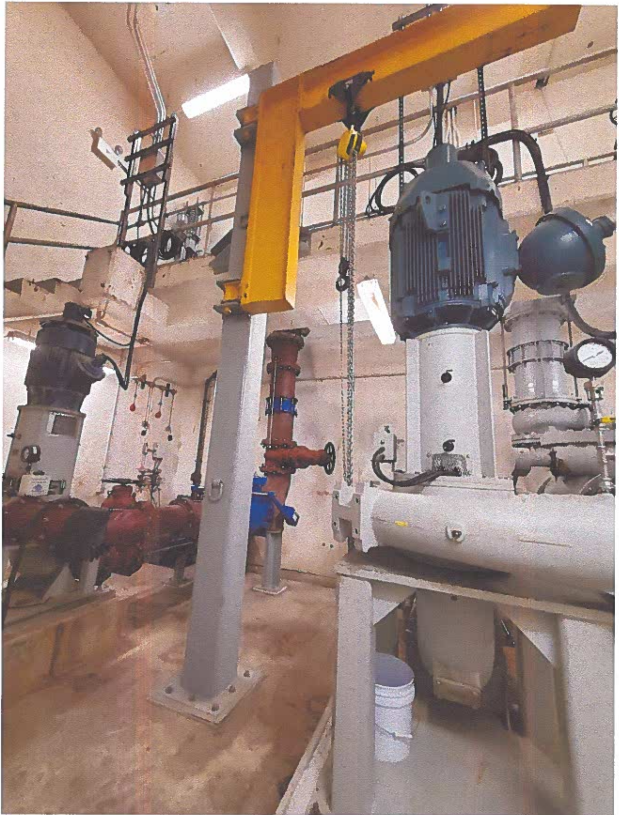
Phase one of the installation
