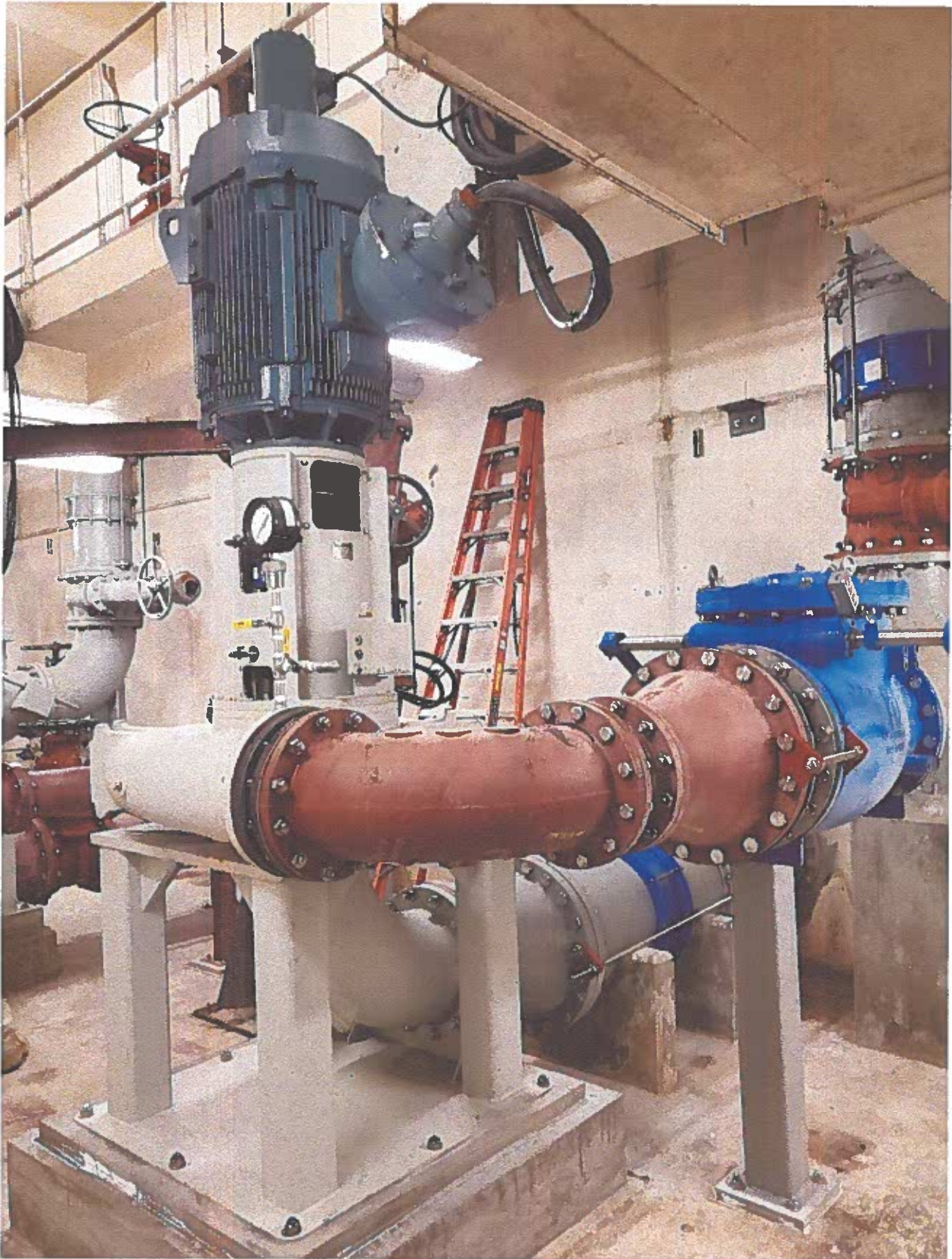
Phase 2 of the Installation #1 large pump
