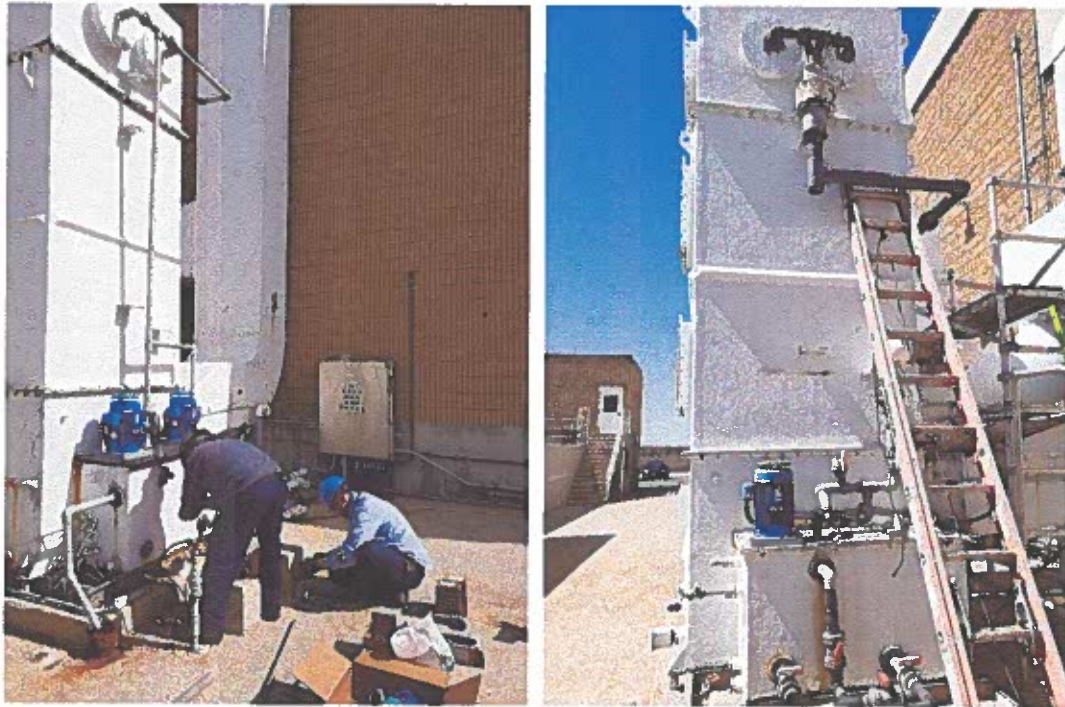
Wildwood/Lower Region Operations Crew installing new piping to scrubber water lines
