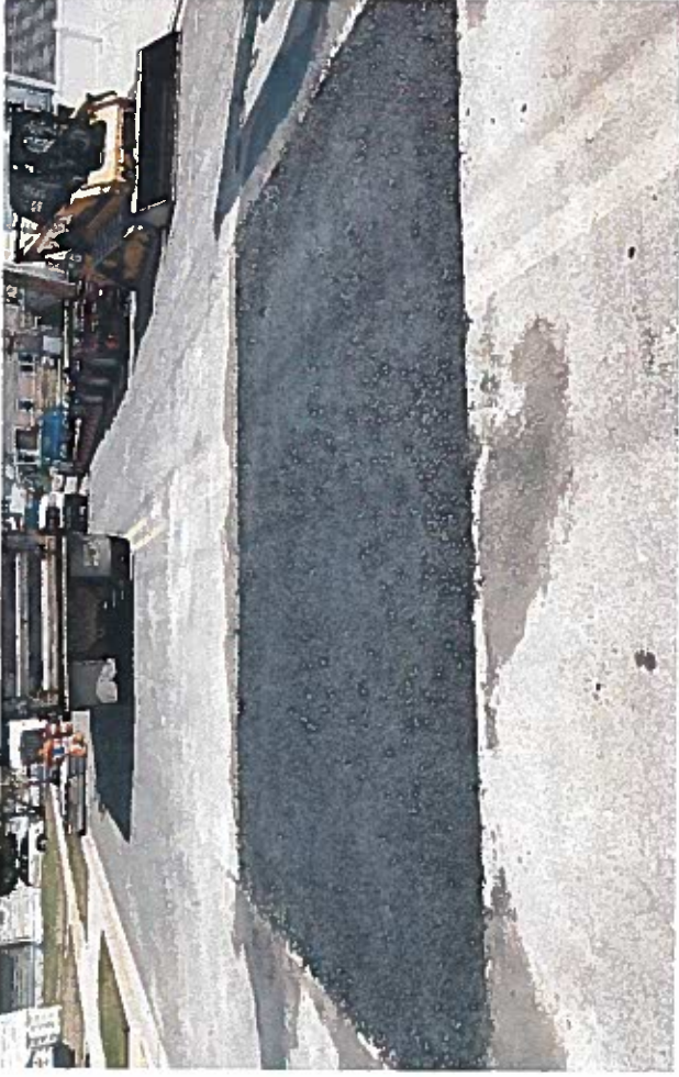
Temporary pavement restoration on Delaware Avenue, North Wildwood (4-11-22)
