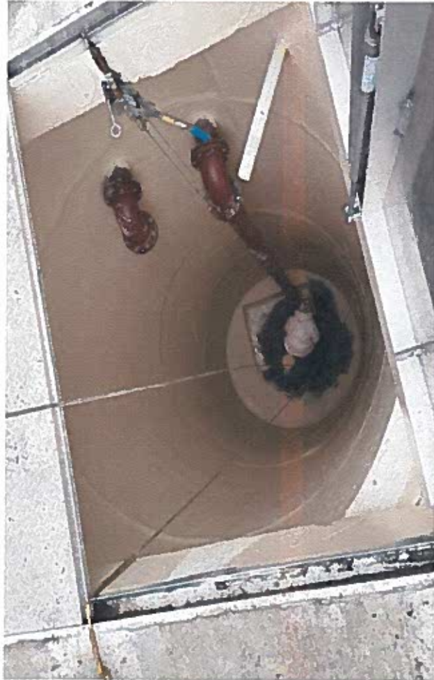
Core drilling for new piping into existing wet well (4-1-22)
