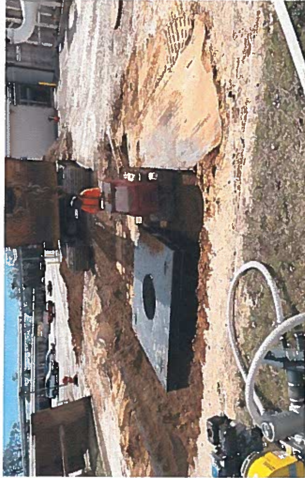
Setting potable water valve (4-4-22)
