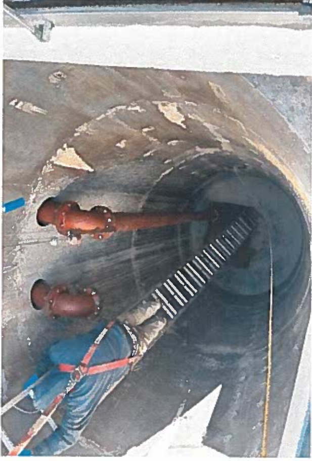
Installing new piping within wet well (4-4-22)
