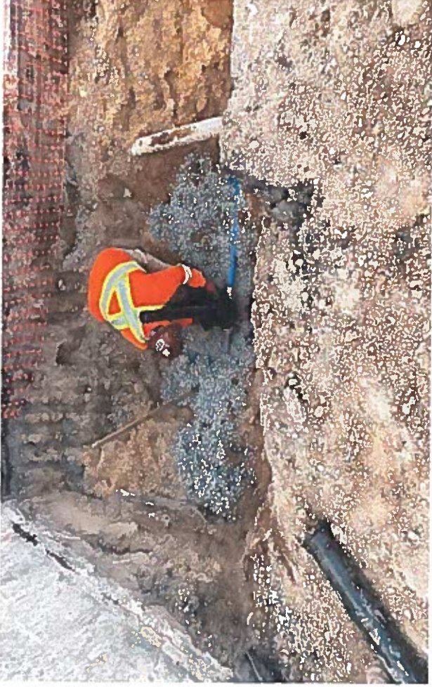
Setting potable water valve (4-4-22)
