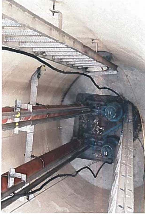
Installing new piping within wet well (4-4-22)
