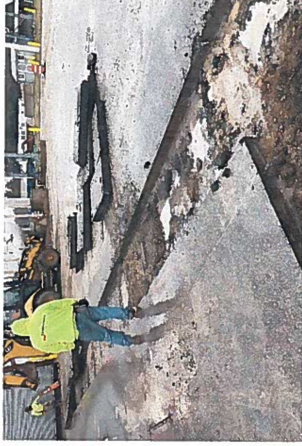
Cutting pavement for trench work (4-6-22)
