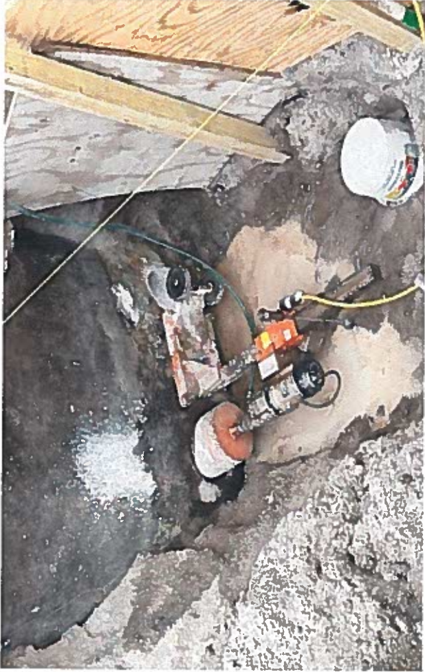
Core drilling for new piping into existing wet well (4-1-22)
