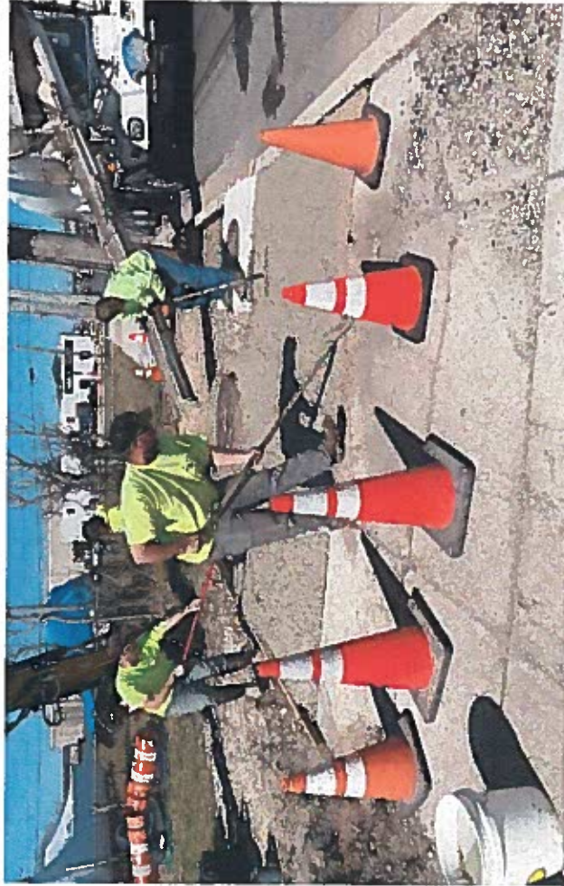
Temporary pavement restoration on Delaware Avenue, North Wildwood (4-11-22)
