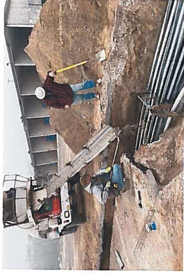
Encasing conduit in concrete (5-4-22)
