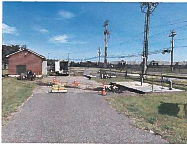
New underground conduits at Crest Haven Pump Station
