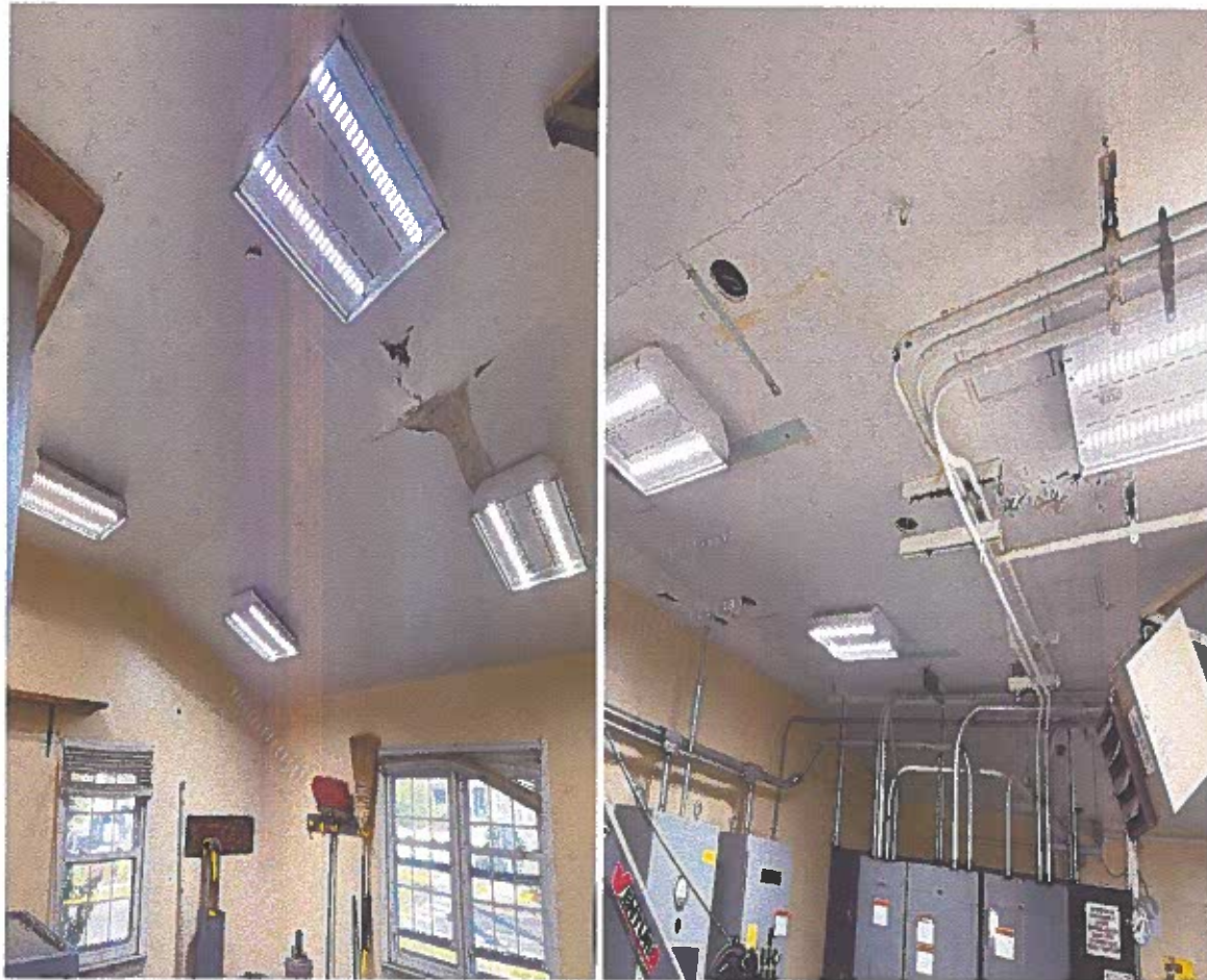
20th St pump station lighting upgrades
