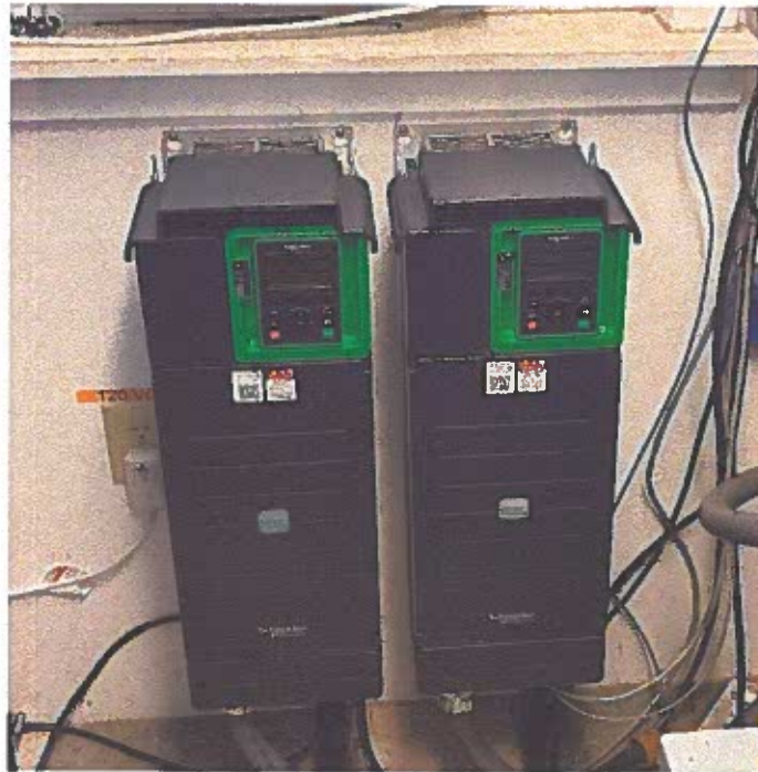
46th St Pump Station VFD Installation
