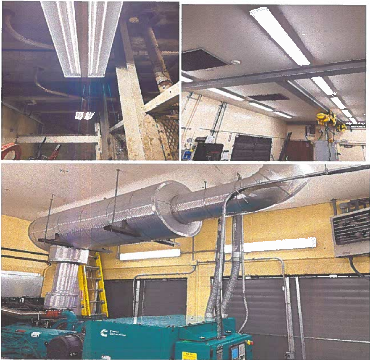
3rd St pump station lighting upgrades
