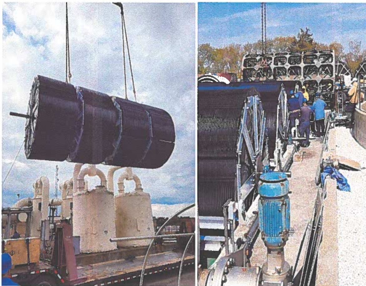
New RBC shafts installed
