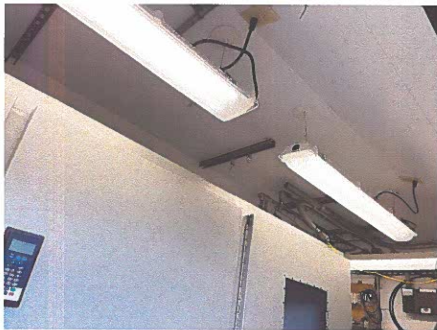
46th St pump station lighting upgrades
