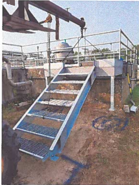
SM/M Scum Pit Platform Installation
