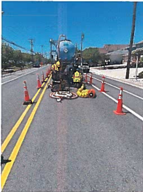
22nd Street air release (left) and leaking air release at 9th Street prior to replacement (right)
