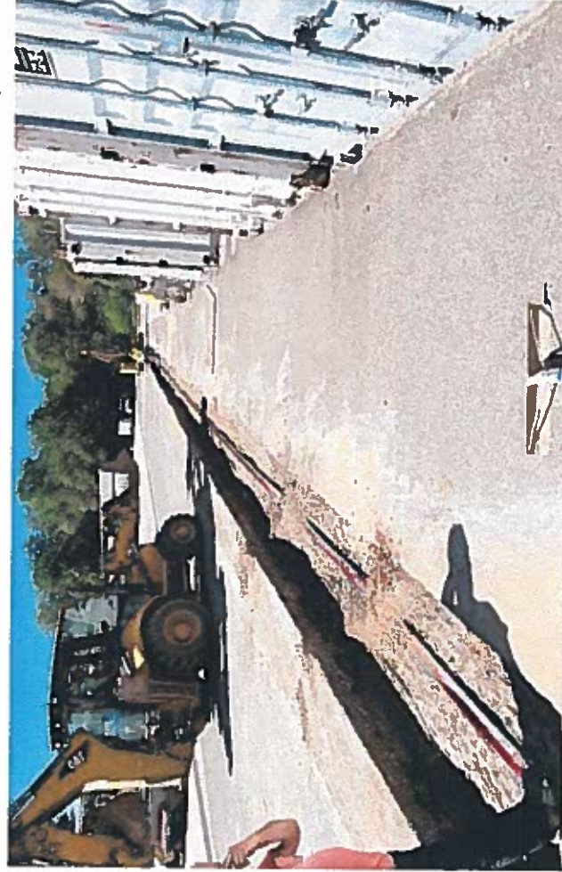
Conduit leading to Electrical Control Building (5-27-22)
