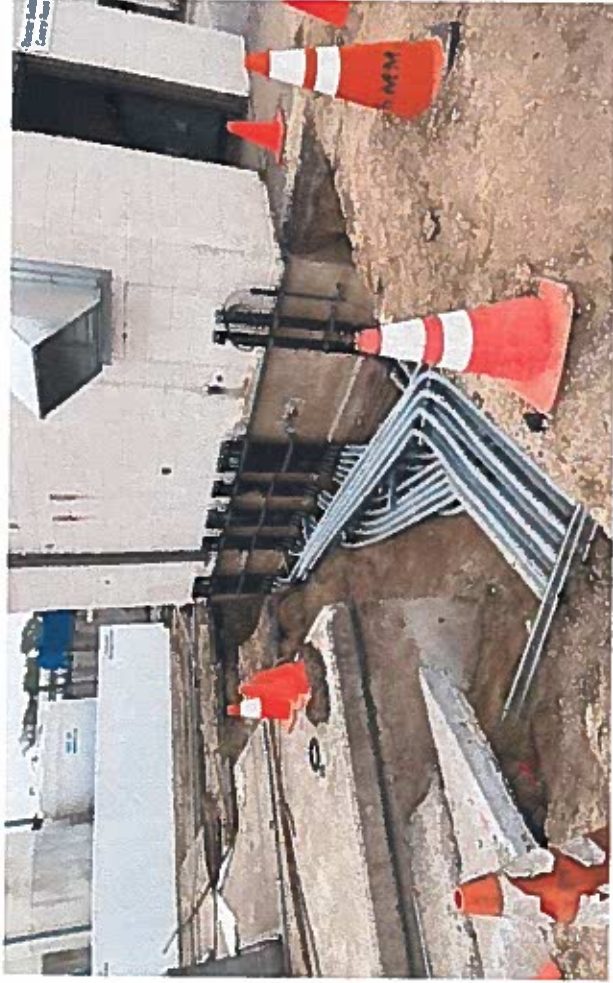
Conduit leading to Electrical Control Building (5-27-22)
