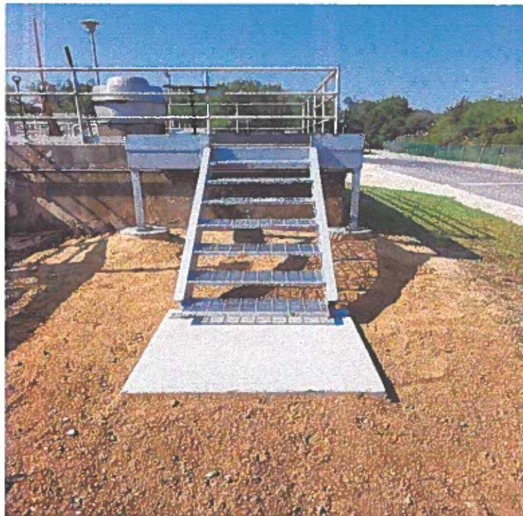
SMM scum pit access stairs
