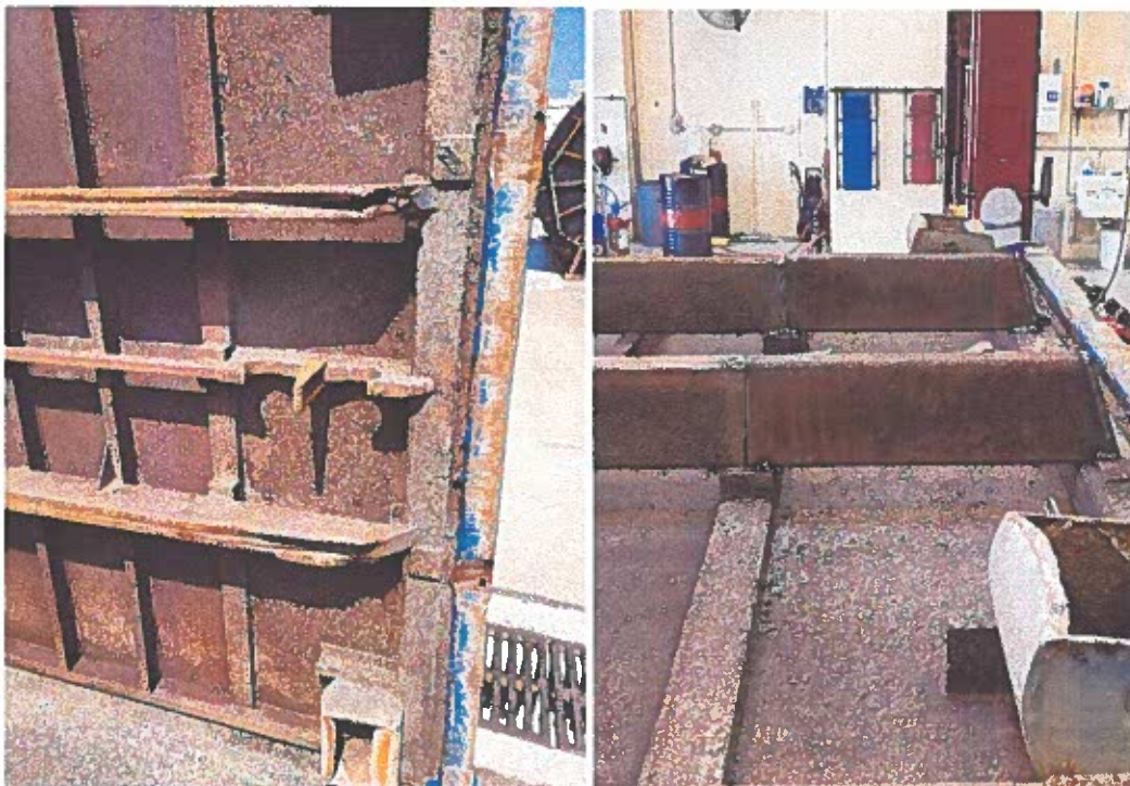
Sludge can rail repairs
