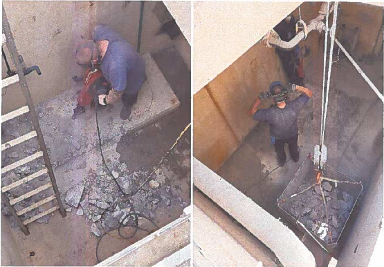
SMM scum pit curb demolition
