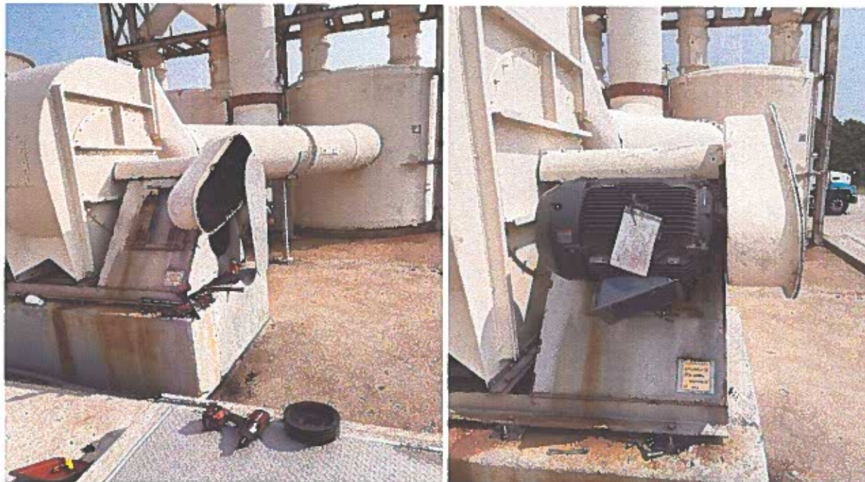
OC Sludge Processing Scrubber Motor Repairs
