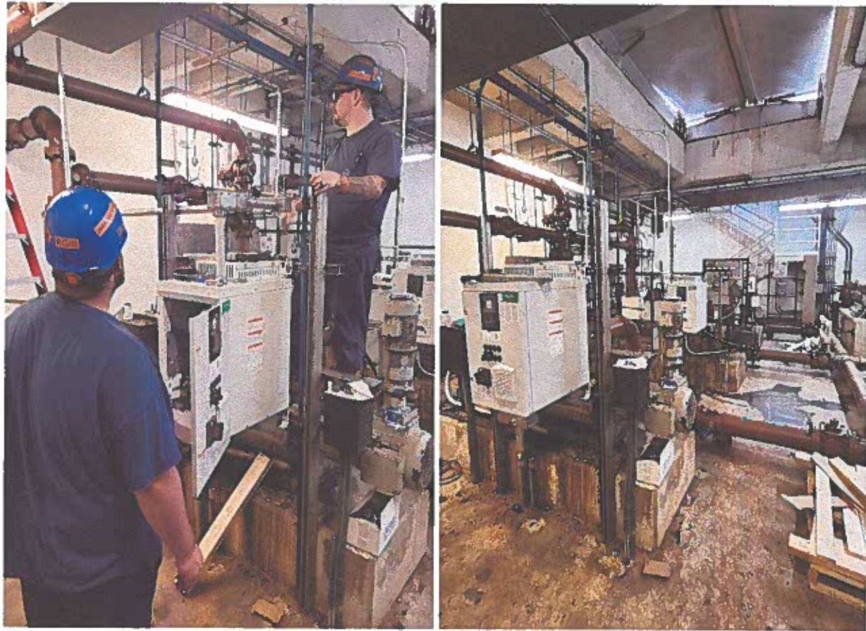
WWL thickener gallery VFD install
