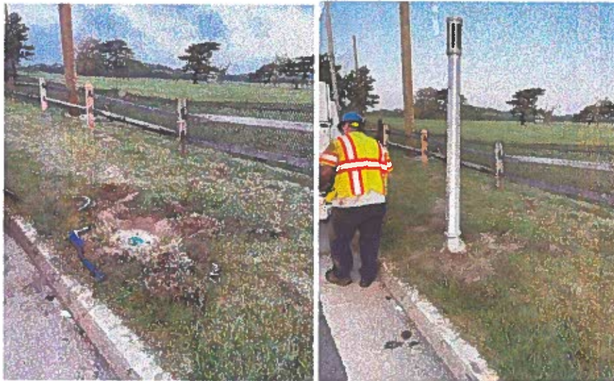
OC air release chamber vent replacement
