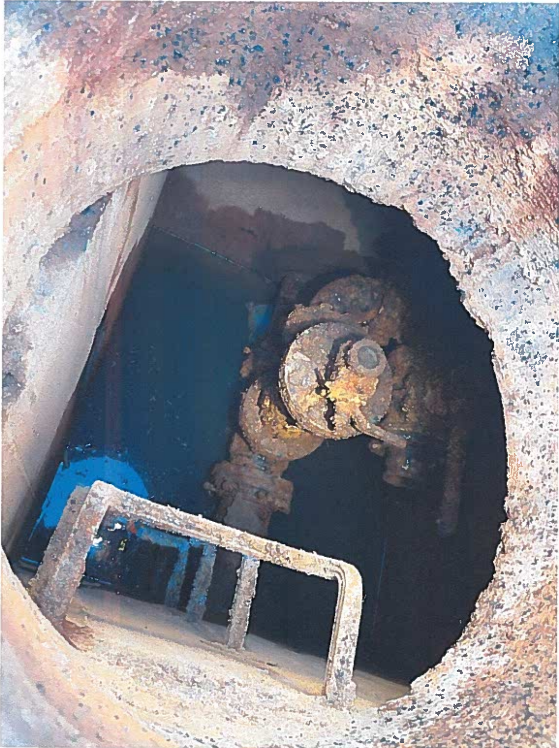
Clean out Chamber
