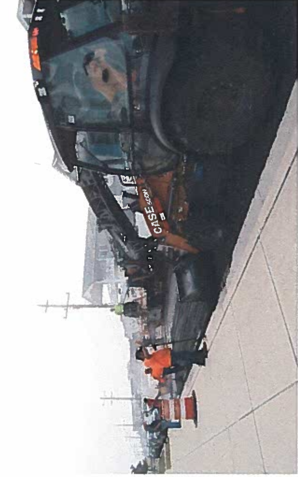
Milling pavement at 14 th Avenue (8-23-22)
