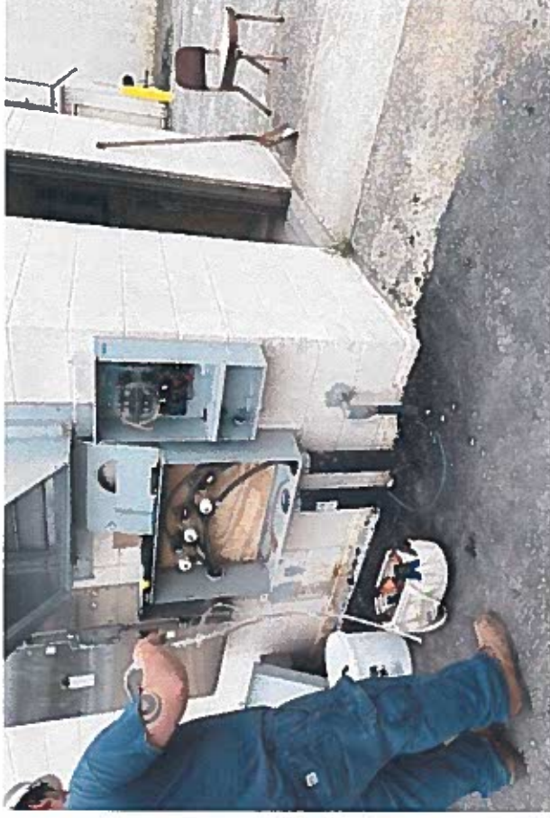
Wiring up new meter at the Electrical Control Building (8-1-22)
